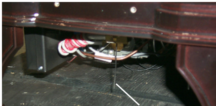
Pull adjustment wire up to close or down to open aeration
